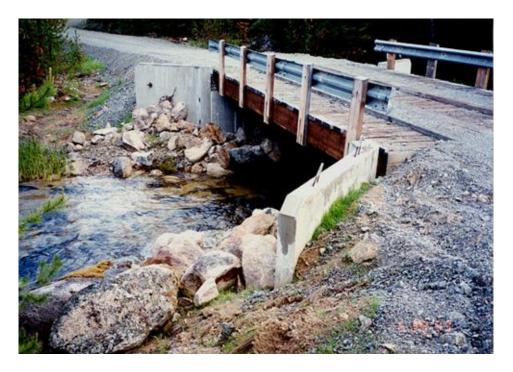
Bridges are best for large stream and those plagued with floatable debris or ice jam problems. Bridges have the least impact on fish.
