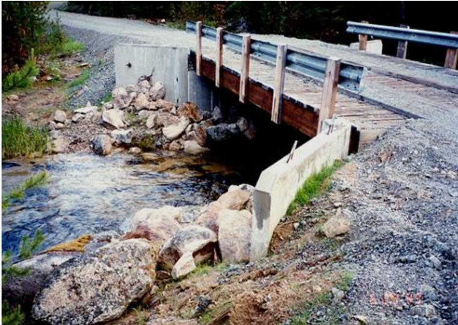
Bridges are best for large stream and those plagued with floatable debris or ice jam problems. Bridges have the least impact on fish.
