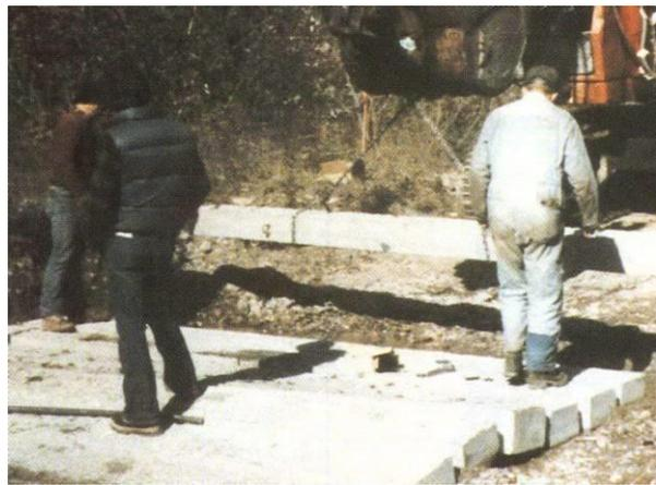
Armoring the streambed and banks with rock, or concrete planks fastened together can provide an improved ford crossing.
